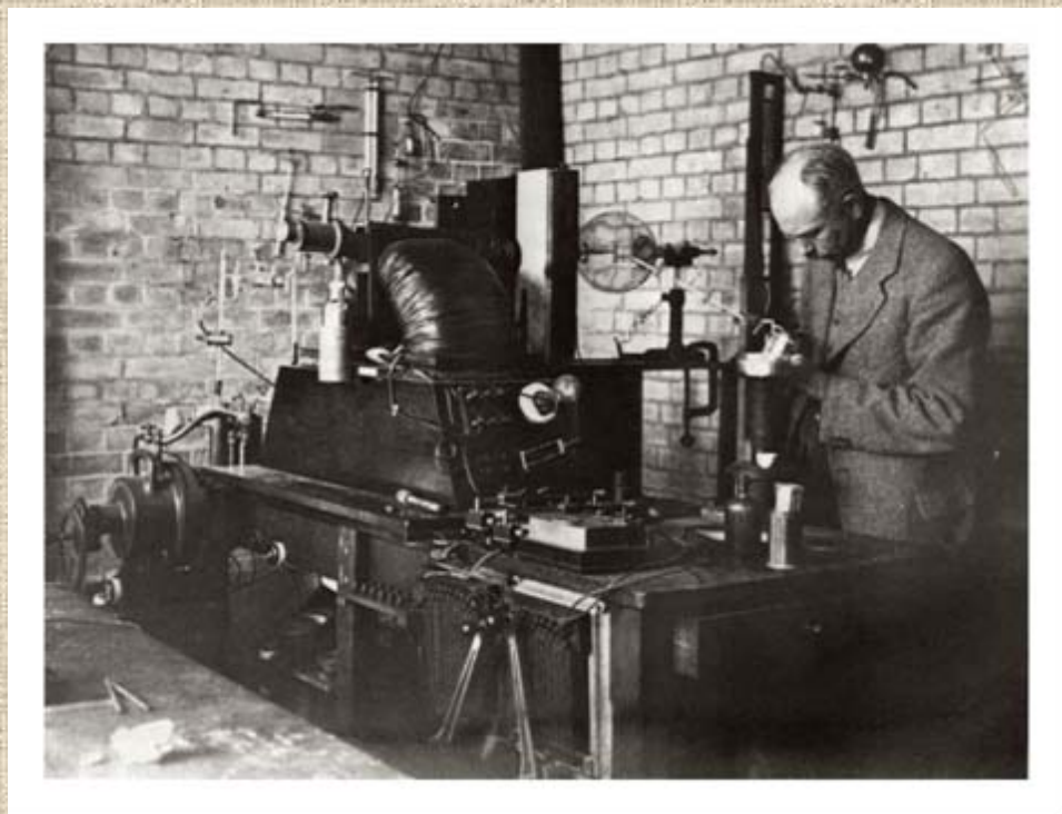
Francis Aston (1877-1945) with his mass spectrograph at the Cavendish laboratory
